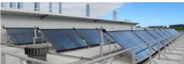
900 solar collector tubes used for water heating.
