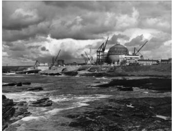
Dounreay Fast Reactor, North of Scotland
